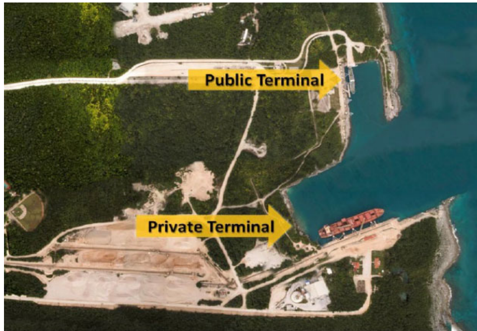
Picture 3 –Aerial View of CALICA’s Port Terminal
