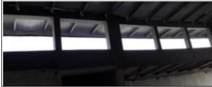
Inspection Report on the “Luces del Pacifico” Residential Project dated 2 Sep. 2019 (C-0031) p. 17, Figure 4
