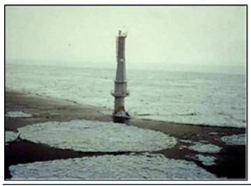
Figure 3.8: Ice action at Yamachiche Light Pier, St. Lawrence Seaway, Canada<sup>20</sup>
