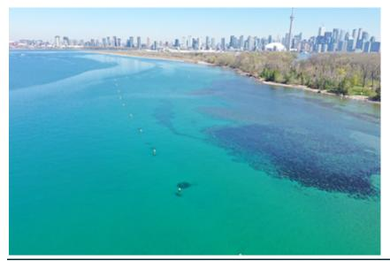
Figure 4.13: Gibraltar Point submerged reef at Toronto Islands created by dumping stone material into Lake Ontario
