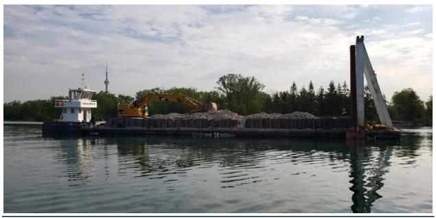
Figure 4.14: Placing stone into Lake Ontario at Gibraltar Point, Toronto Islands
