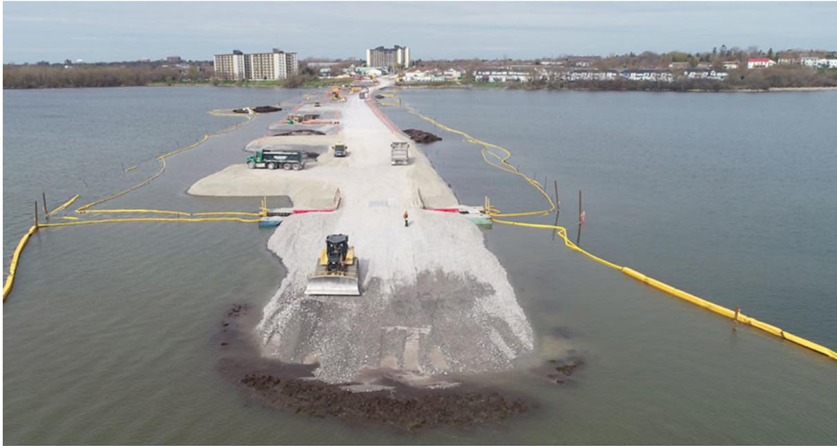
**Figure A.71 - Third Crossing Construction Using a Temporary Causeway Across the Cataraqui River, Involves Dumping Fill Material in Provincially Significant Wetland, 5km Directly Upstream of Water Intake**
