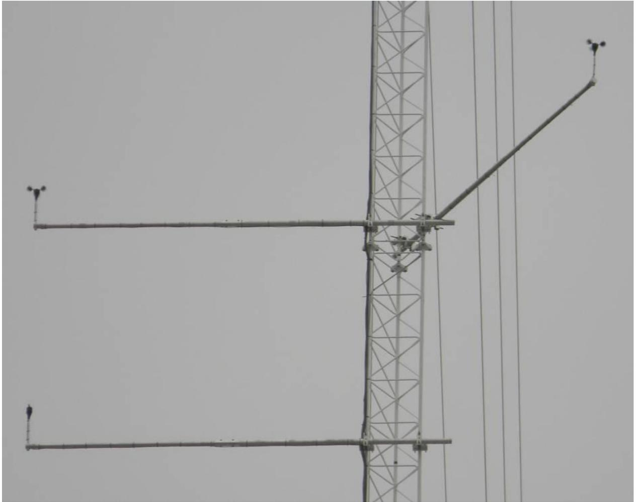
**Figure A.9 - Instruments at Levels 6 and 7**
