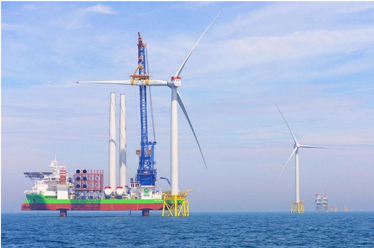
**Figure 8 – Turbine Installation at East Anglia ONE<sup>85</sup>**
