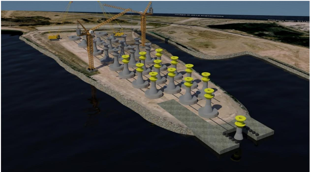
**Figure A.32 - Fabrication Facility with Foundation in Launch Position**
