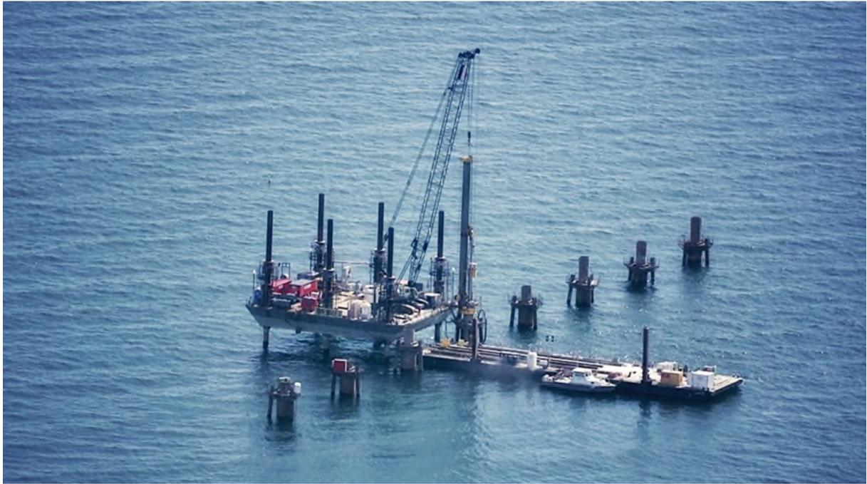
**Figure A.68 - Marine Construction of In-lake Risers for Ashbridge's Bay Treatment Plant Outfall Project, Lake Ontario**
