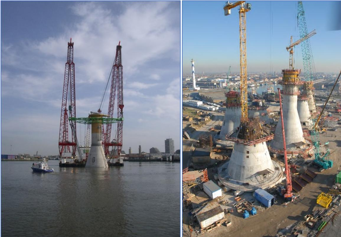
**Figure A.28 - Thornton Bank Offshore Wind Farm GBF Under Construction, February 2008**
